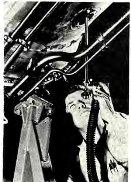
Inside inspection using a Anvar quartz-rod endoscope
